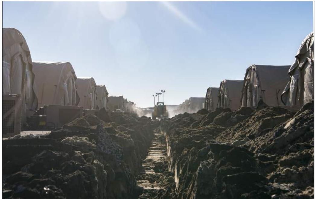
Civil engineering Airmen from the 23rd Civil Engineering Squadron, Moody Air Force Base, Ga., dig trenches through tent city for laying more permanent high-voltage power lines at Tyndall Oct. 28. Support personnel from Tyndall and other bases are working to repair base infrastructure and build bare-bones facilities after Hurricane Michael. *Air Force photo by Airman 1st Class Kelly Walker*
